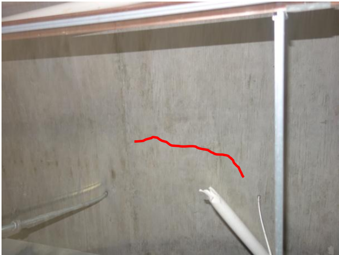
顶板横向裂缝1条,缝长1m,最大缝宽0.12mm
