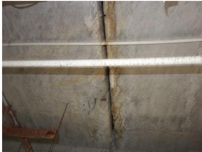
顶板砼掉块露筋,面积S=0.25*0.4m²
